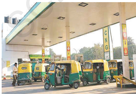
Fig - 3: CNG gas filling station
